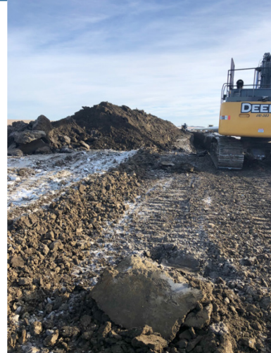
2. Excavator and spill pile – Km 144+200 – Jan 8, 2018
