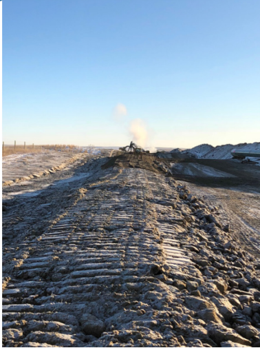
13. Backfill – Km 159+700 – Jan 11, 2018
