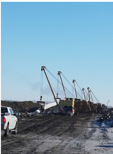
17. Track hoe cleaning clumps in ditch-162+600 - Jan 12, 2018
