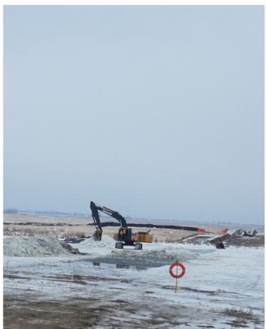
5. Track hoe (wetland) – Km 165+050 – Jan 9, 2018
