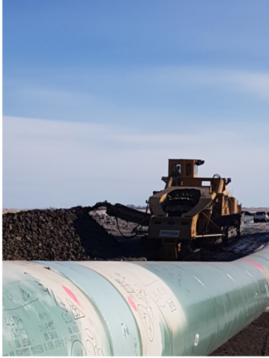
19. Excavators digging out plug - km164+850 – Jan 13, 2018
