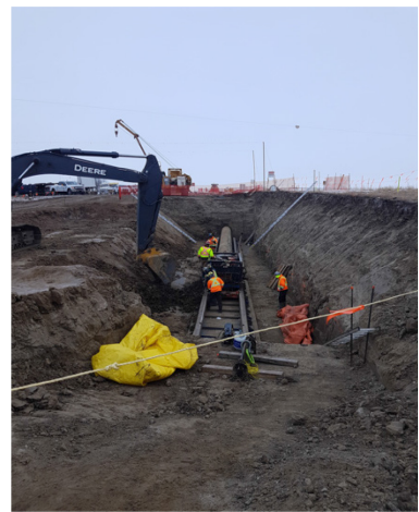
6. Spill Piles - Km 163+500 – Jan 9, 2018
