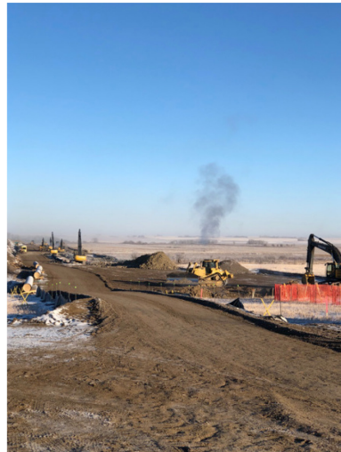
16. Bore crew and dozer at bore pit – km 161+000 – Jan 12, 2018
