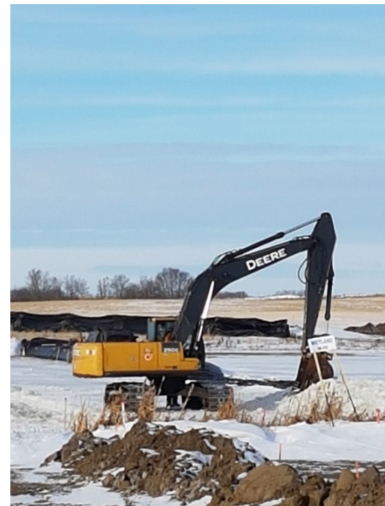
4. Track hoe working on wetland - Km 165+300 – Jan 8, 2018
