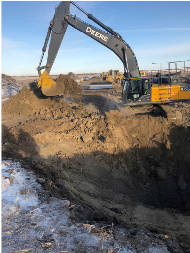
21. Excavator digging in bore bay – Km 161+000 – Jan 13, 2018
